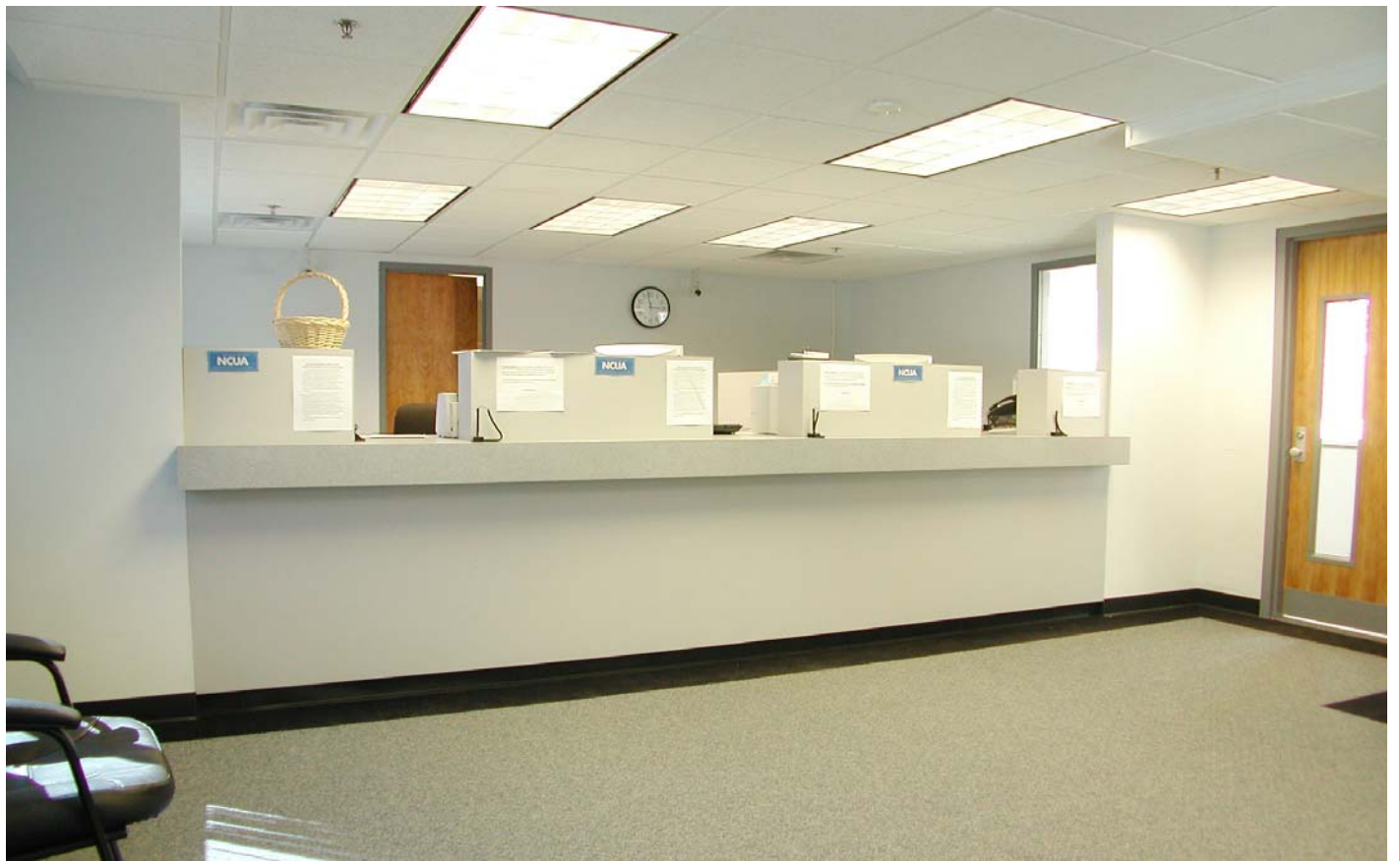
TYPICAL SPACE AFTER RENOVATION
