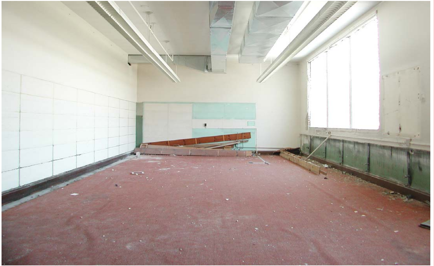
TYPICAL SPACE BEFORE RENOVATION
